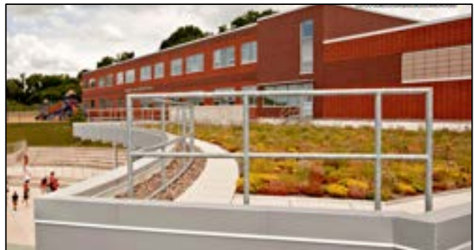
Selinsgrove Elementary School – Selinsgrove, PA
