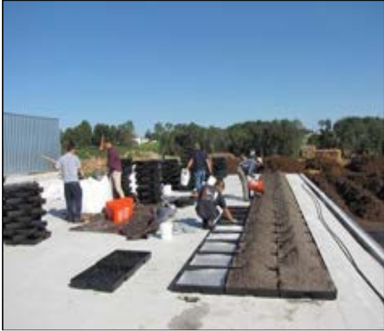
Green Roof under construction at Laurel Valley Farms
